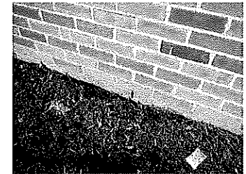
Photo 12 Weeps at grade along south elevation.
