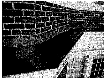
Photo 15 EPDM installed over wood cornice elements of 1927 Building.
