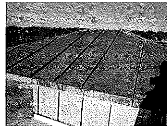
Photo 17 Standing seam metal roof at vent.
