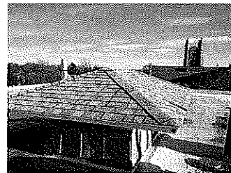
Photo 18 Asphalt shingle roof at vent.
