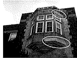
Photo 1 Cast stone elements above east entrance. Patches are circled in yellow. Efflorescence and surface staining typical at joints. Mortar repair at parapet (red arrow).
