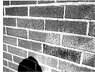
Photo 10 Typical brick masonry condition at 1950s addition.
